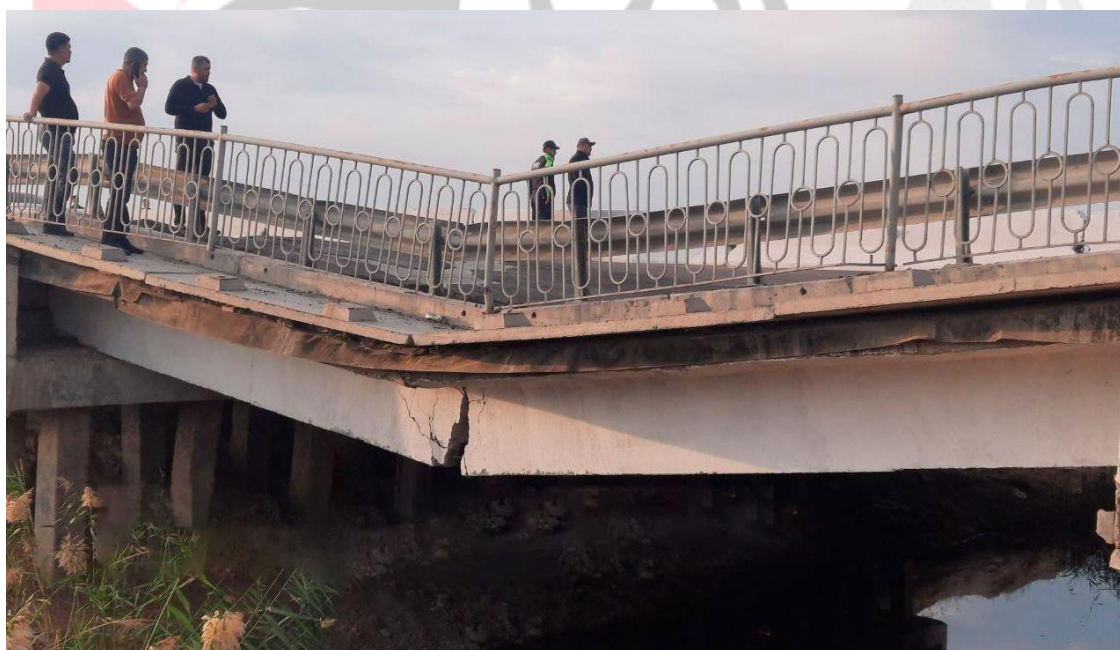
Picture 1. In the Akaltin district of the Syrdarya region, a bridge broke and the road collapsed.
