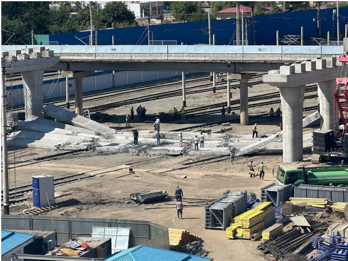
Picture 2. Five beams of an overpass under construction near the airport in Tashkent collapsed.
