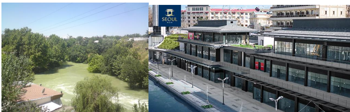
Fig. 11, 12 Burjar Canal embankment (before and after reconstruction)
