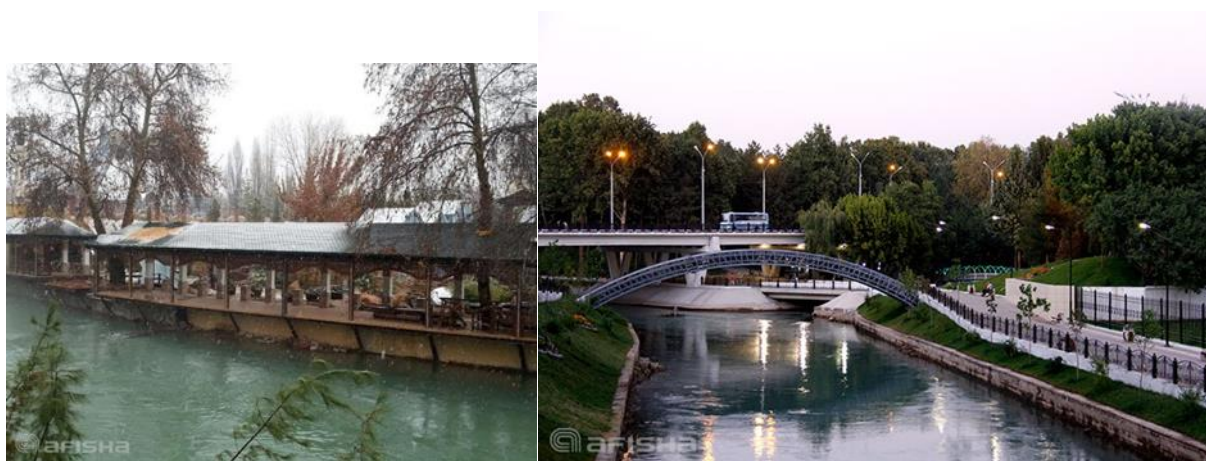
Pic. 13, 14 The Anhor embankment before and after reconstruction.
