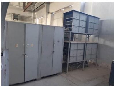
Figure 1. Distribution cabinet with load resistance
