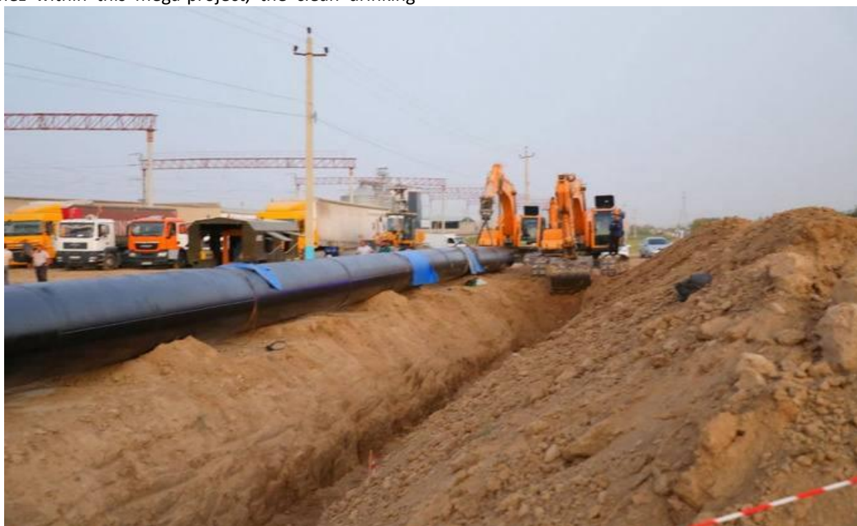
Figure 4. Construction process of the main water network from the Topolon reservoir to the city of Termez in the region.
