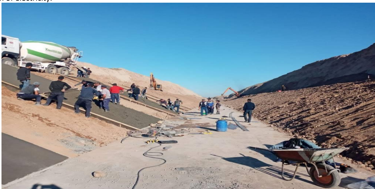
Figure 2. Repair process of the Khazarbog' - Oqqapchig'oy canals.
